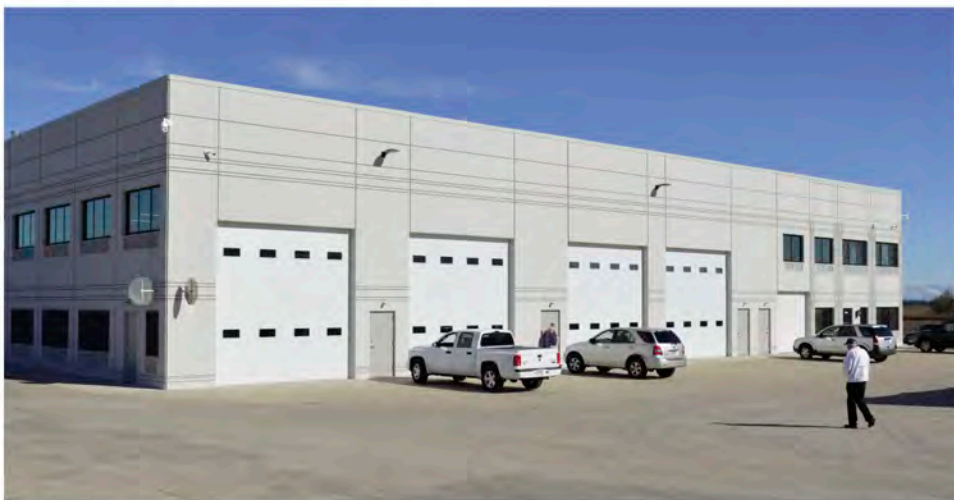
The landlord envisioned Grand Craft's facility as a distribution center with natural light, four large garage doors on one side and two more on the opposite side.
